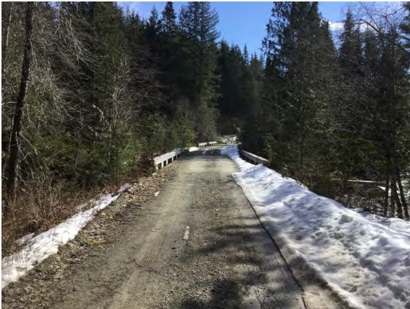
Approach from Right Bank when facing downstream
