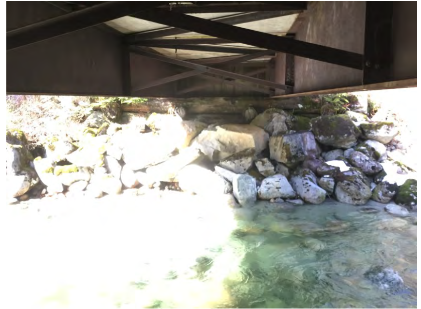
Right Bank Abutment when facing downstream
