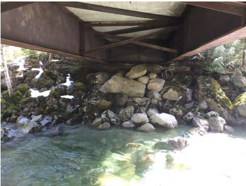
Left Bank Abutment when facing downstream
