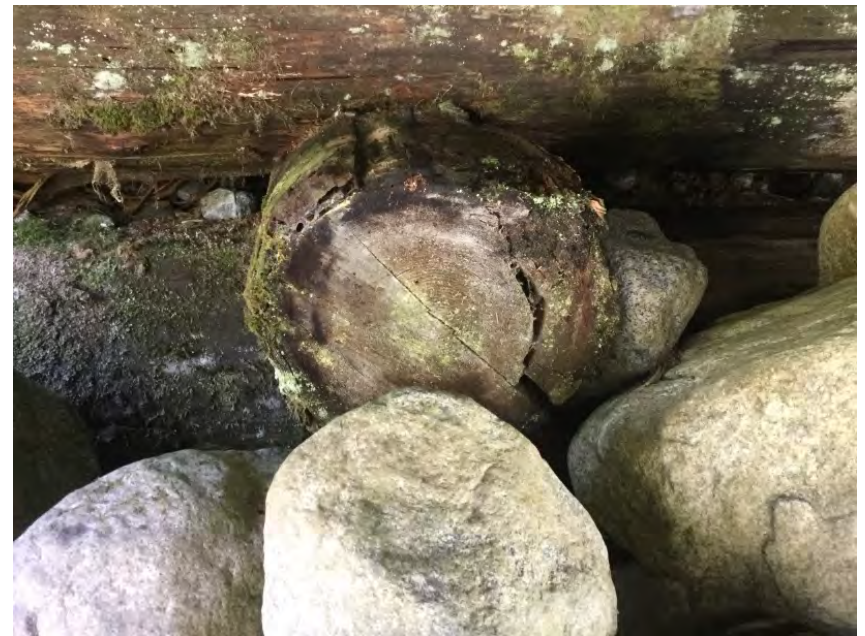
Tieback condition, typical
